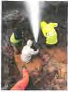
Employees work to repair a water main break.
